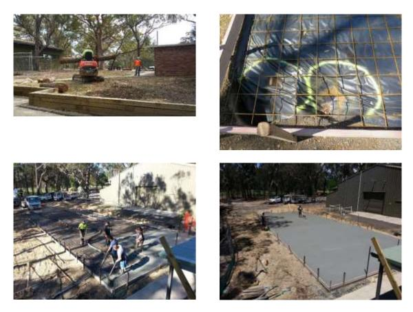
Work on new building is finally progressing. Safety fencing has been installed and sediment control installed, trees felled, stumps ground, roots removed, site levelled with excavator, western berms created to stop run-off, waste water drainage exposed, plumbing and storm drainage planned with quotes obtained
