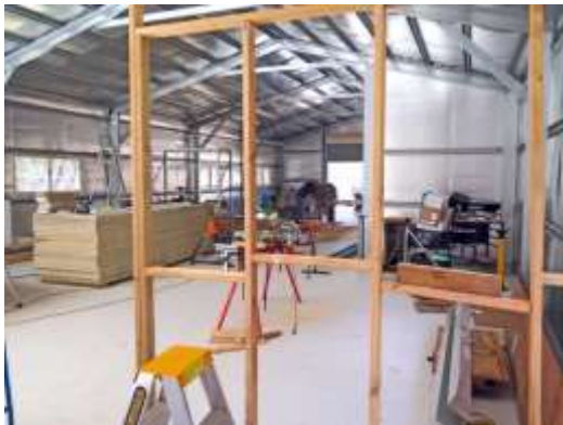
Partitions are underway Wall lining boards are in the background
