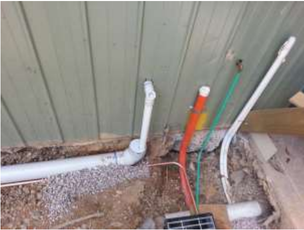
New outlet for metalwork sink gravity drainage
